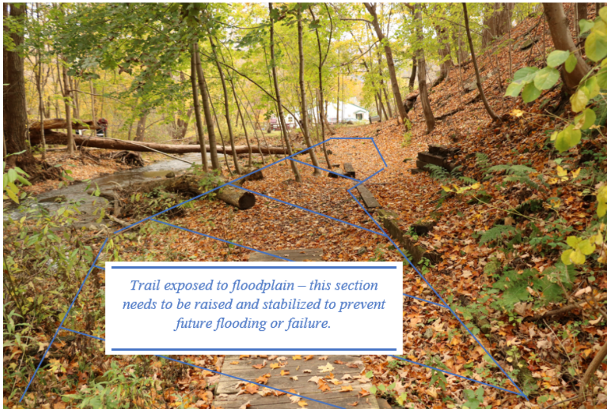
Figure 16: Exposed Trail with Floodplain outlined (blue)
