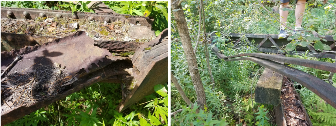
Figure 7. Burke No. 25, 66.5 ft-span
